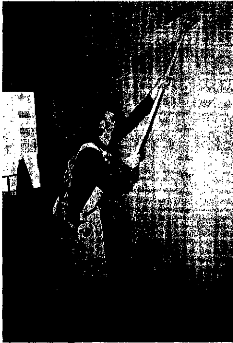
Figure 1 — Pole sanding of drywall taping compounds. Several applications of taping compounds may be required to make a smooth joint between gypsum wall boards, requiring extensive sanding.
